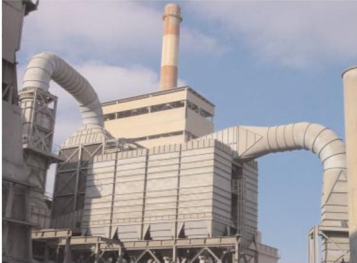
Electrostatic baghouse for collecting particulates at a cement plant.
