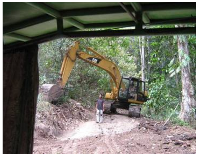
Road Building Lembata, Indonesia
