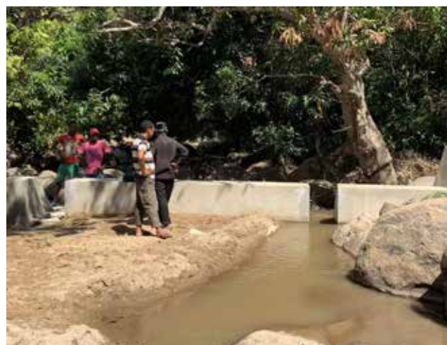
4) Damming of a stream
