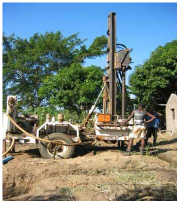
2) Drilling for ground water
