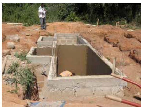
A building with 6 toilets will be built above the pit
