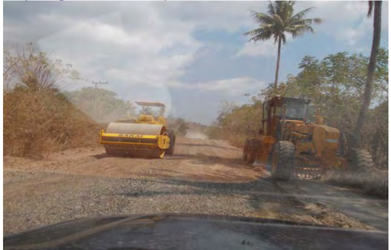
Preparing the road for asphalt
