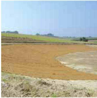
Application of GREENFIX Eromat for a detention reservoir (during installation)
