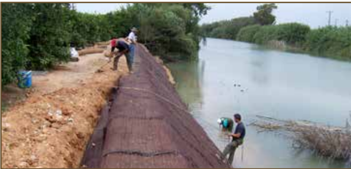
14.1 Shoreline protection with GREENFIX 75-C
