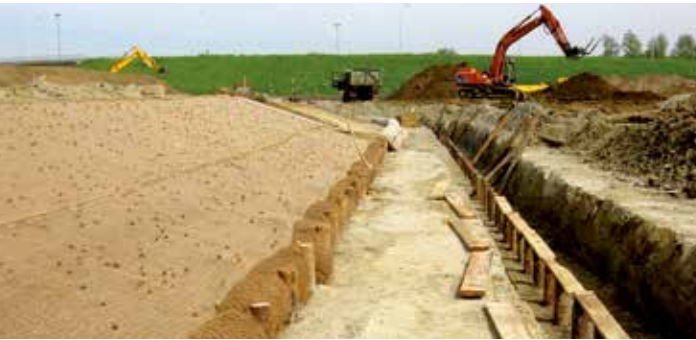
Enviromental friendly solution with Covamat fresh and Bio-Logs
