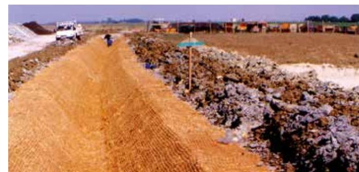
Protection of a road side channel with Covamat plus
