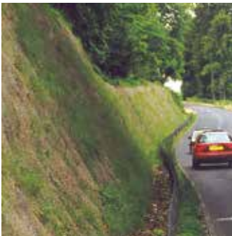
Erosion protected slope after six weeks
