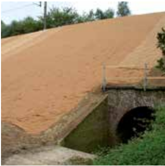
Slope protection with GREENFIX Eromat on a steep rail-road slope
