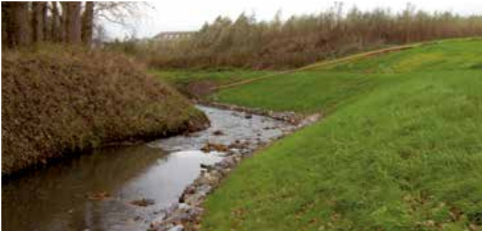
Protection of the embankment through grass establishment
