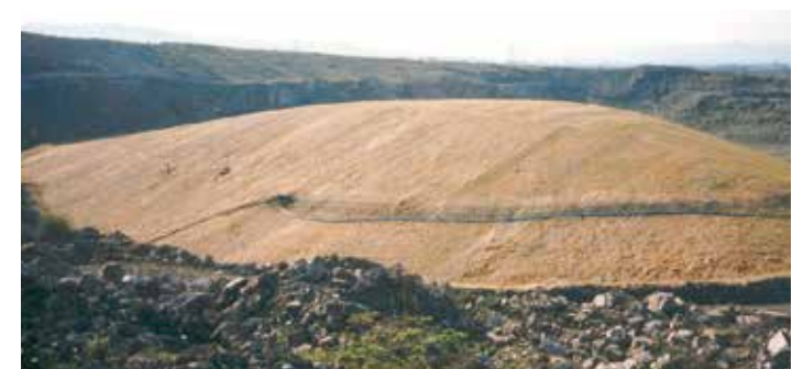
Ready installed Covamat plus on a landfill job for temporary erosion protection
