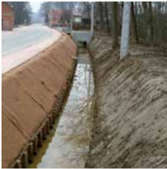
Slope protection along a surface drain with GREENFIX Eromat
