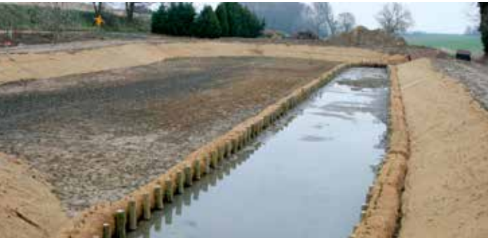
The Bio-Logs were delivered with plant holes for quick insertion of water plants
