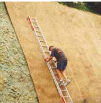
GREENFIX Rockmat Type 5D installation on 65° steep slope
