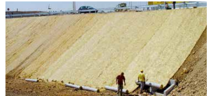
Motorway slope protection with Covamat plus in Lisbon/ Portugal
