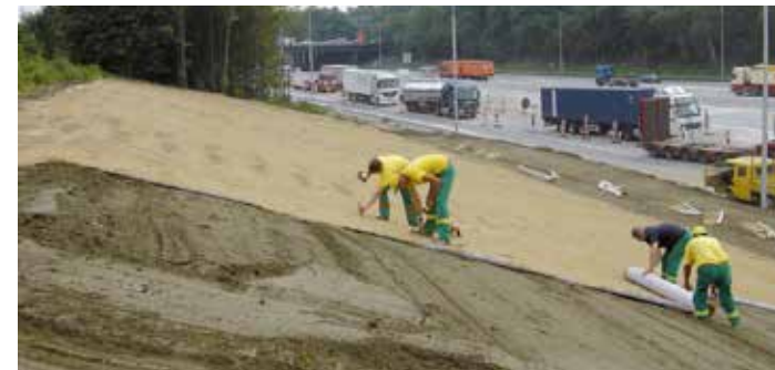
Approx. 60.000 sqm of Covamat fresh have been installed at the ring road of Antwerp/ Belgium
