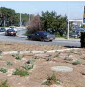
Plant protection on a traffic island with GREENFIX f³ Mulchmat in the South of France.
