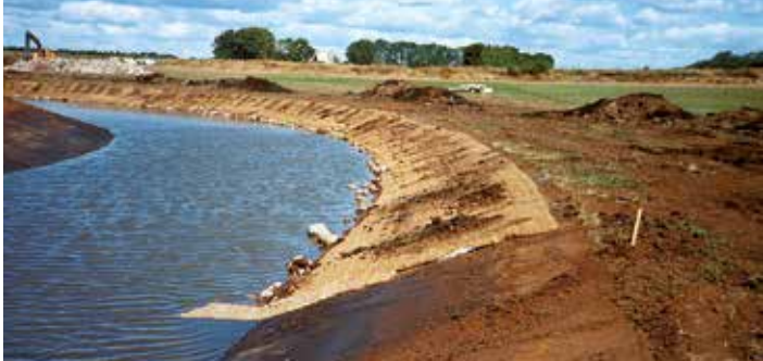
The use of Covamat plus with biodegradable nettings
