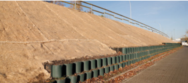
SoilWeb® Geocells and GREENFIX® Erosion Control Blankets
