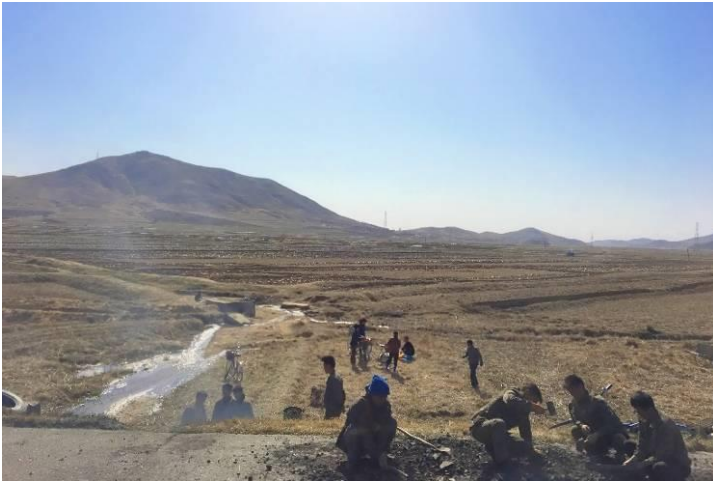
Smashing rocks with basic tools to repair road
